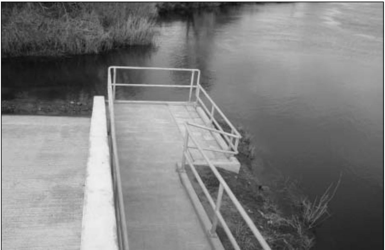
A newly constructed facility for disabled anglers on the Moy at Foxford, Co. Mayo
